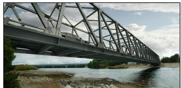
Fig 1 Steel Truss Bridge
